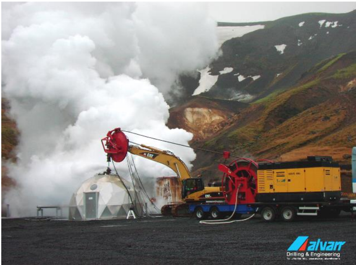
Soft starting a HiTemp well in Hellisheidi near Reykjavik - Iceland, in late 2009.
